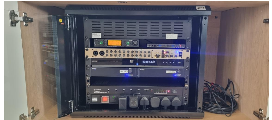
Example Hall AV System installed at Dunblane Cathedral including BluRay and Loop Amplifier
